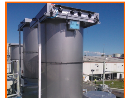
New reverse-jet filters fitted
