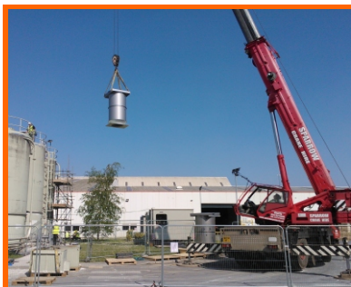
Complete project installation
