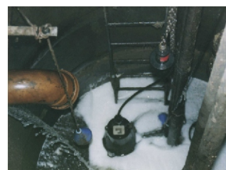
Sewers and drains which are inaccessible for foam detection
